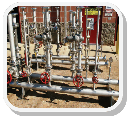
Completed manifolds undergoing hydrostatic pressure test.
